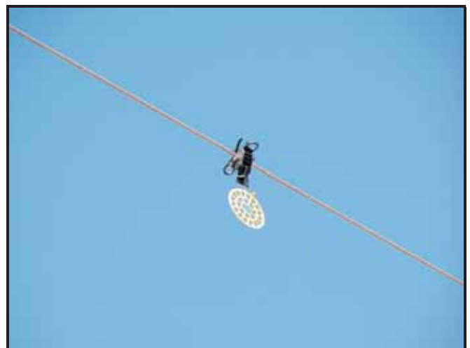
Figure 4: A "Bird Flapper" device which is attached to the overhead conductor and moves with the wind.
